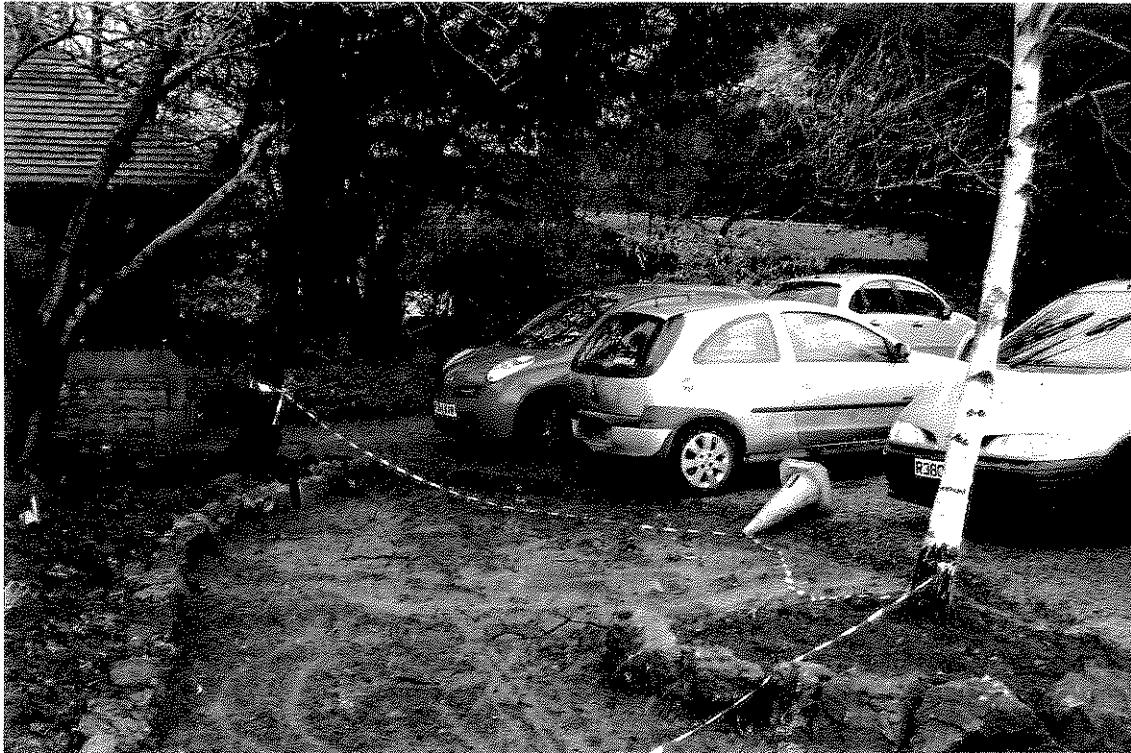
Recent development works + exposed damaged roots, to front of St. Johns Church,
